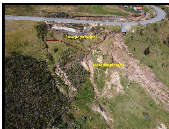
Figura 75. Deslizamiento 1. x: 744810,226; y: 9657952,441; z:2834,61
