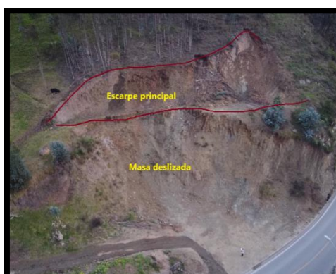
Figura 87. Deslizamiento 13. x: 745034,970; y: 9661713,744; z: 2401,23
