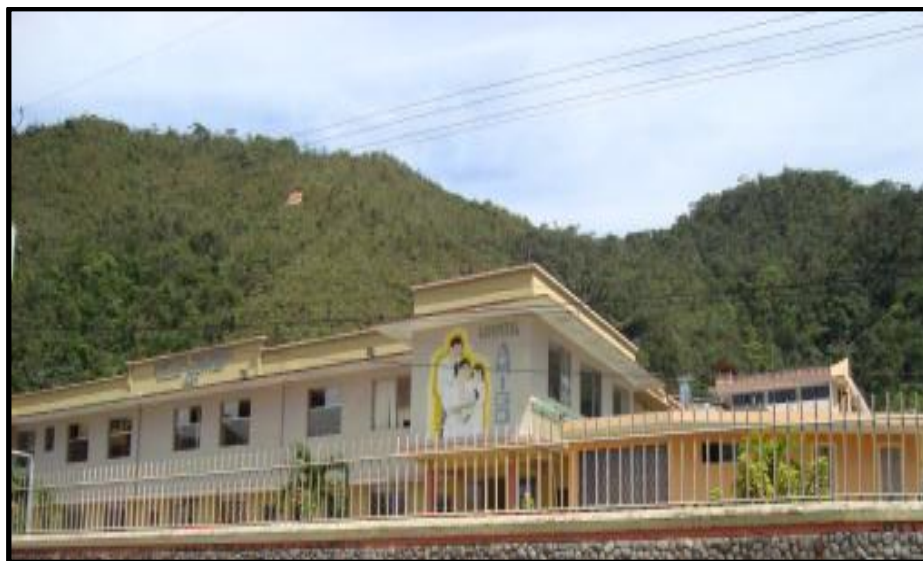
Figura 1. Exterior de hospital Julius Doepfner
